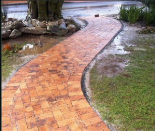
BLOCK PAVING DRIVEWAY
